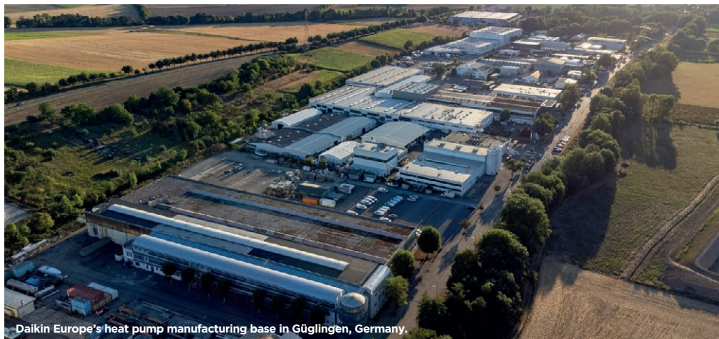
Daikin Europe's heat pump manufacturing base in Göglingen, Germany.
