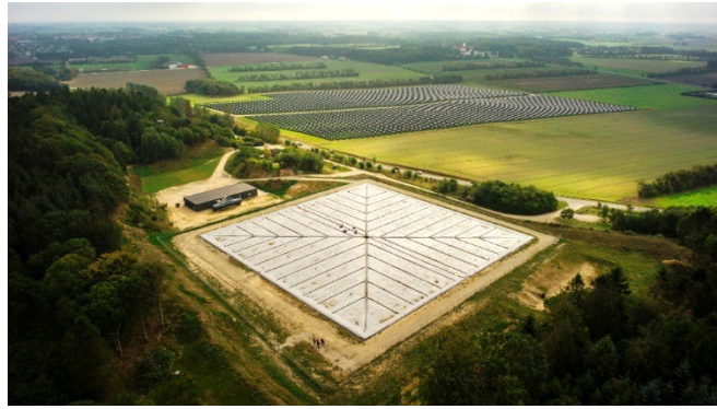
Figure 3. Seasonal thermal energy storage pit at Dronninglund Fjernvarme, Denmark (Epp 2019)
